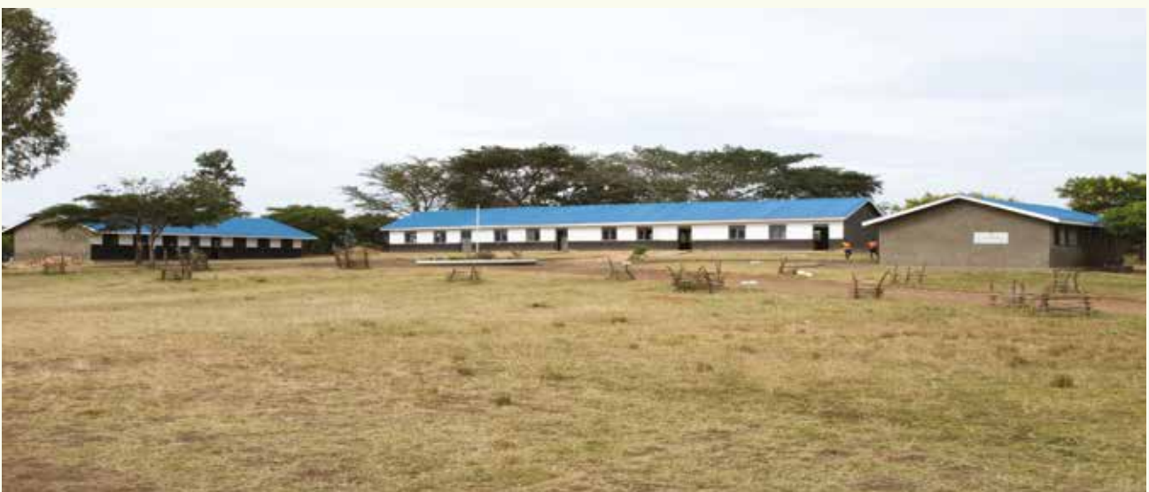
Nama primary school renovation, Gaining Scale training
